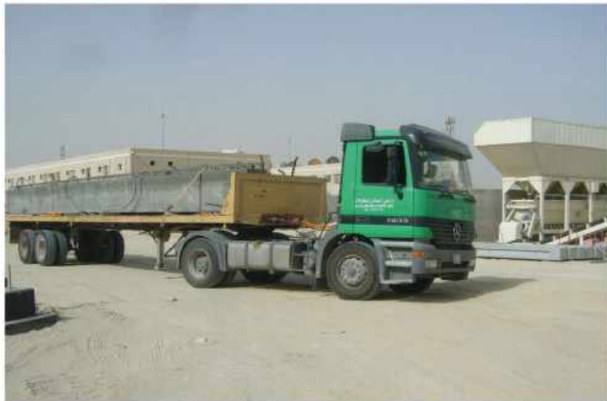
Precast Girder for SRO
