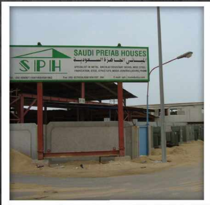
SAUDI PREFAB HOUSES ( BOUNDARY WALL & STAFF ACCOMMODATION )
