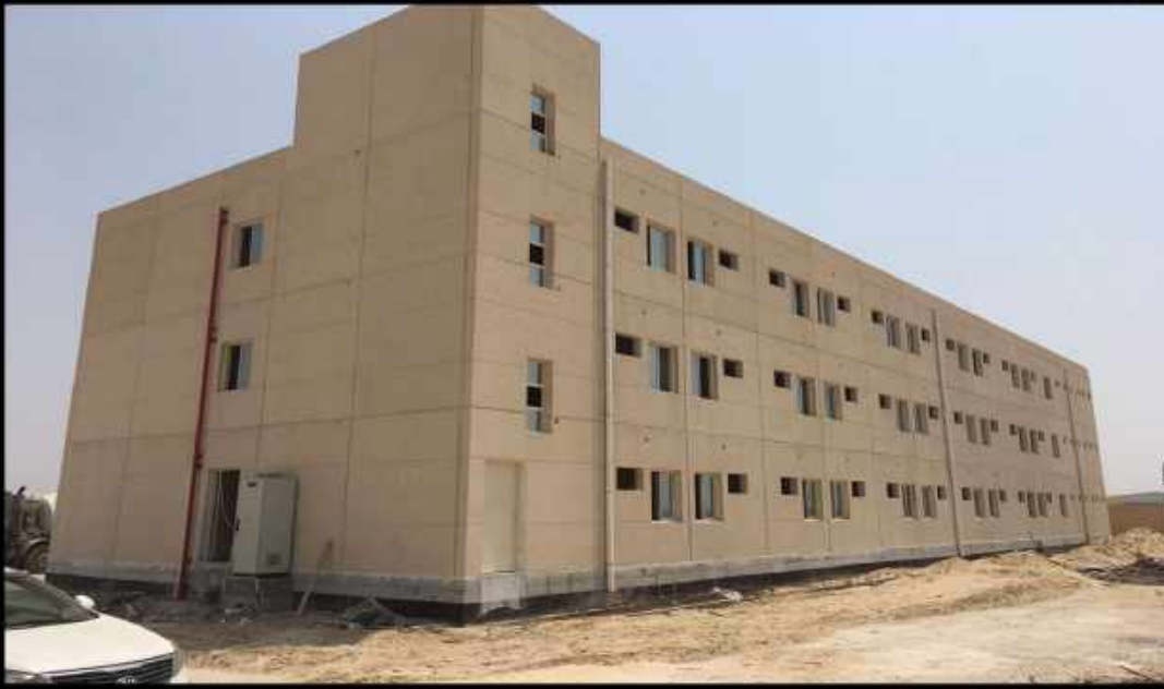
1 UNITS OF 3-STOREY PRECAST LABOR CAMP AL- HOSSAN COMPOUND
